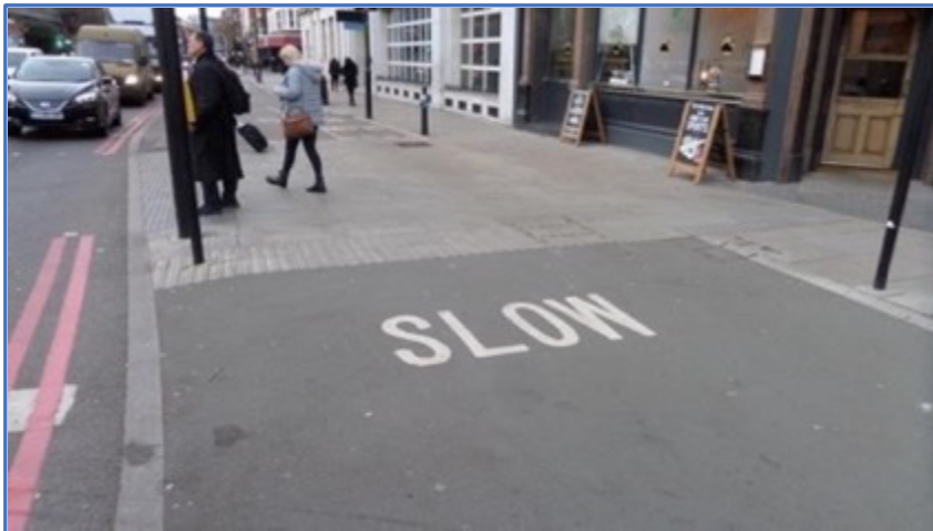
Figure 4.6 Inadequate signage at shared space entry point - cyclists
