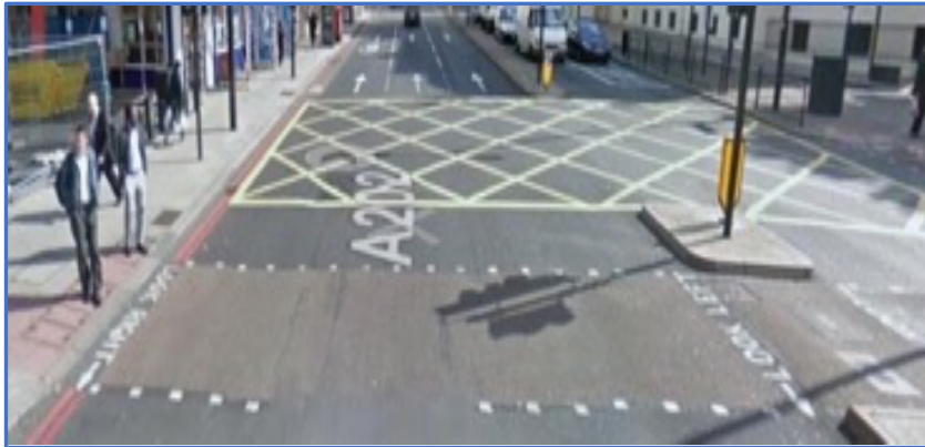
Figure 4.16 Removal of safety affordance – dedicated yellow hatch box
