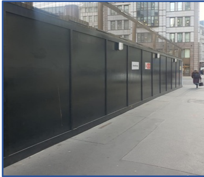
Figure 4.18 Hoardings creating dangers
