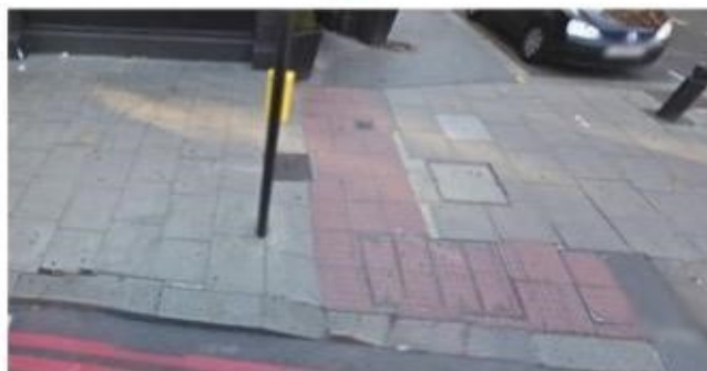
Figure 4.41 Pedestrian crossing point tactile – before and after Shared Space treatment
