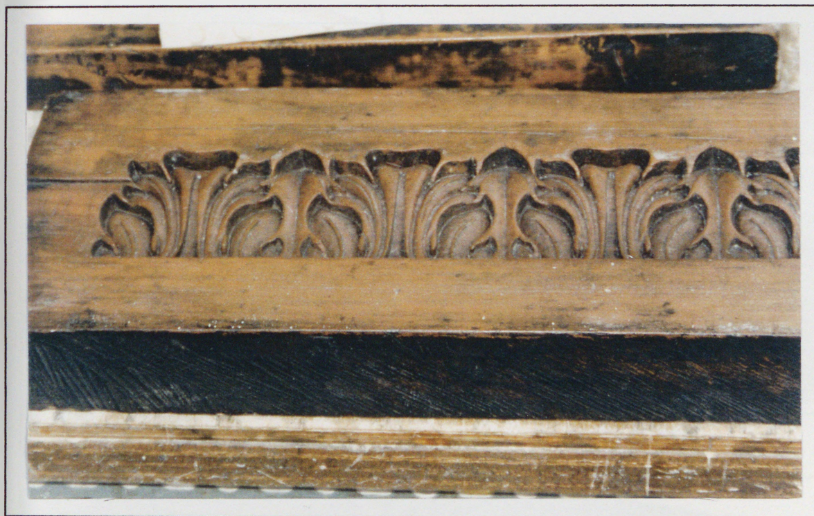
Fig. 41 A mould exhibiting the irregular striations of a hand saw seen here on its edges (Collection of George Jackson & Sons)
