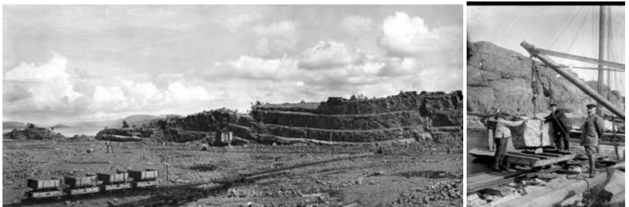
Figure 4.12. Railway on the east side of Langøya. Each carriage could take 7-8 tonnes of limestone. © Slemmestad bibliotek/Cementmuseum/Geologisenter.
