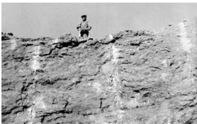
Figure 4.15. Drilling. The limestone quarry had several thin layers of clay which made extraction easier, 1930-40. Vestfold Fylkeskommune © Slemmestad bibliotek/ Cementmuseum/ Geologisenter.
