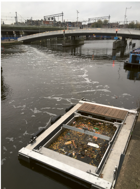
The Great Bubble Barrier catches estuary/river detritus and shepherds it to floating refuse containers. Once clear, the barrier is easily removed from the aquatic location. Credit | The Great Bubble Barrier.
