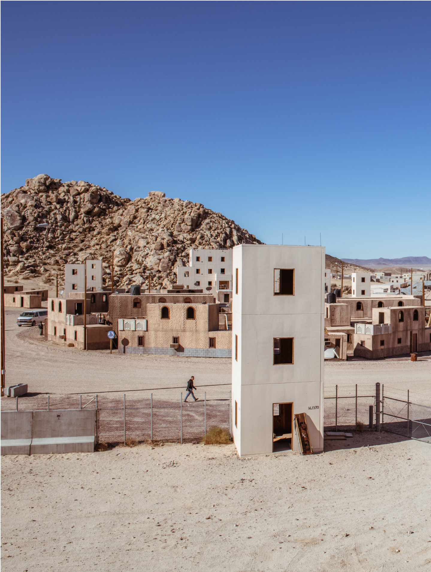
Razish center, view from roof, Fort Irwin NTC, Mojave Desert, California, 2019 © K.Yoland
