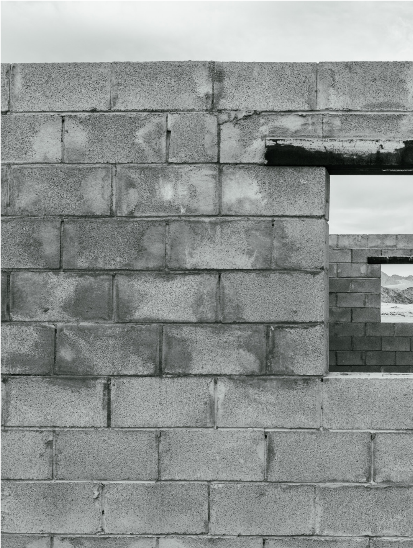
Permenantly half built buildings, Razish, Fort Irwin NTC, Mojave Desert, California, 2019 © K.Yoland
