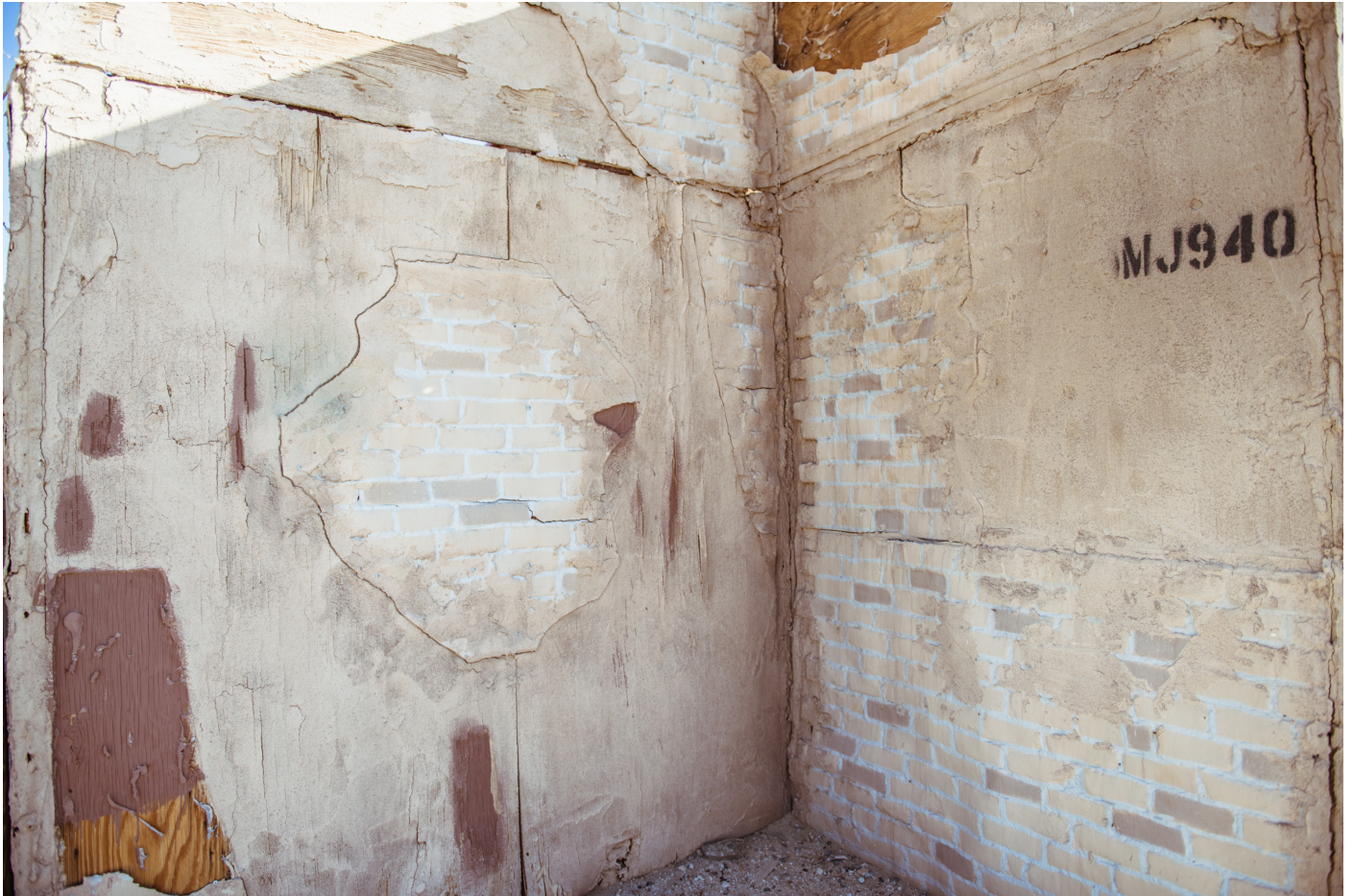
Detail of fake brick work painted onto wood, Fort Irwin NTC, Mojave Desert, California, 2019 © K.Yoland
