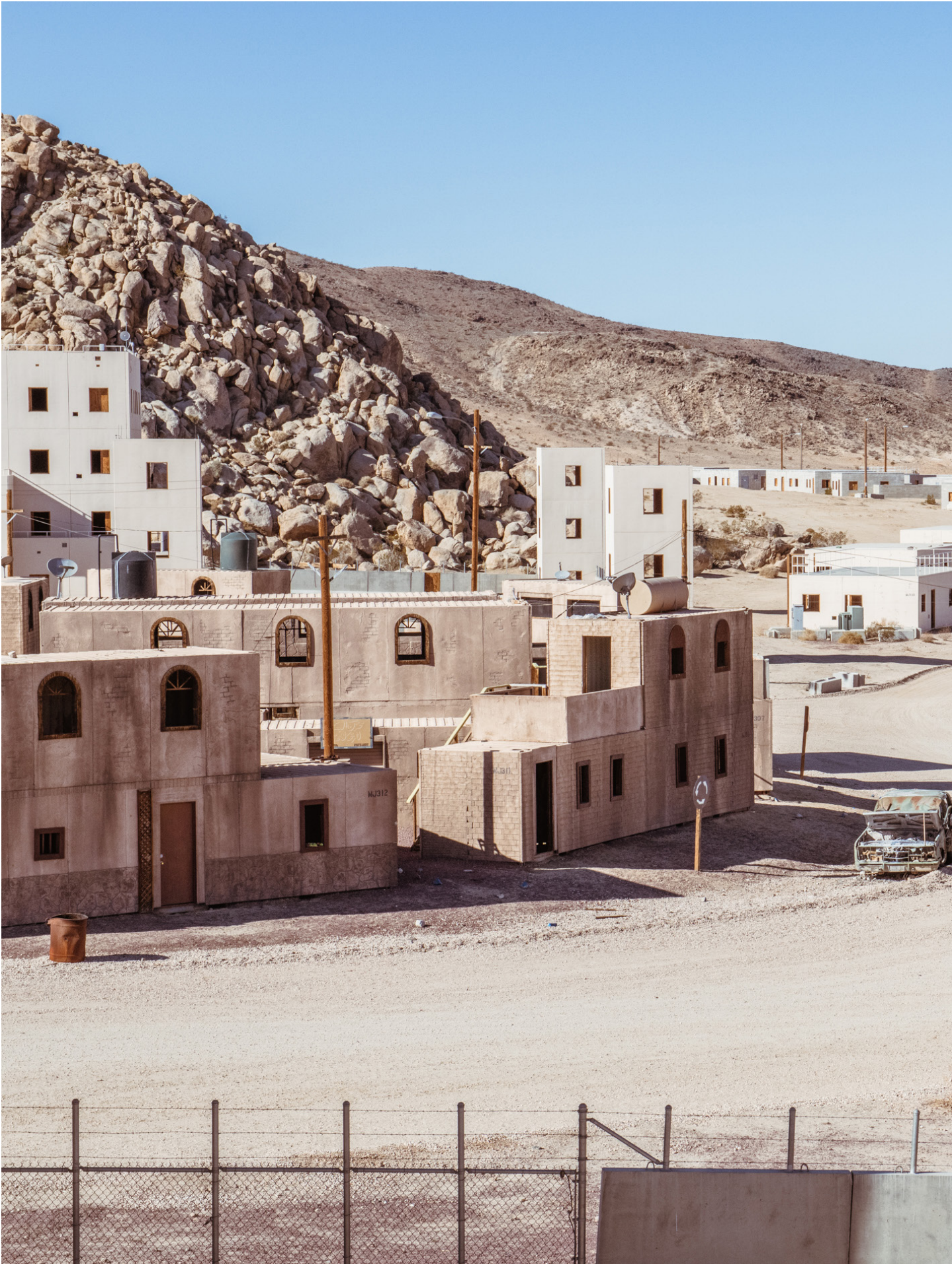
Razish center, view from roof, Fort Irwin NTC, Mojave Desert, California, 2019 © K.Yoland
