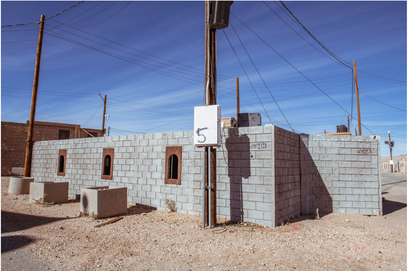
Fake brick work painted onto wood, Fort Irwin NTC, Mojave Desert, California, 2019 © K.Yoland
