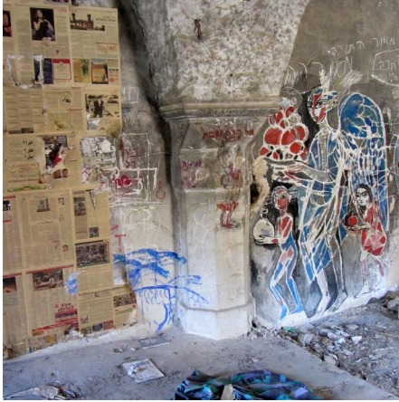
Figure 6. House 68, the octagonal stone column supporting vaults. Courtesy of Riwaq Centre: Lifta documentation project.
