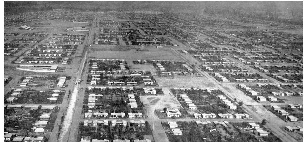
Fig.2 The San Gregorio housing project in Santiago de Chile during the construction phase. Source: Corporación de la Vivienda, Plan habitacional , 99.
