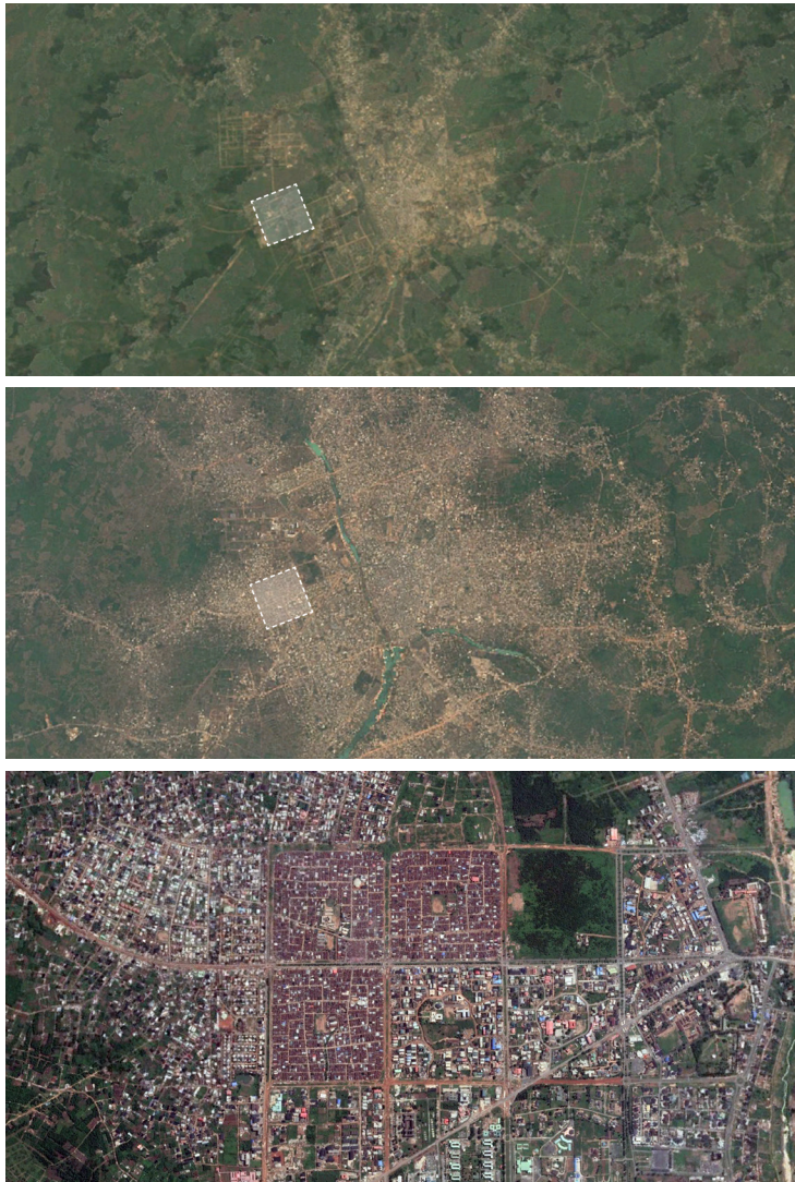
Figs.52-4. Sites and Services project in Owerri, Nigeria in 1985 (top) and 2020 (middle and bottom). Source: Google Earth.
