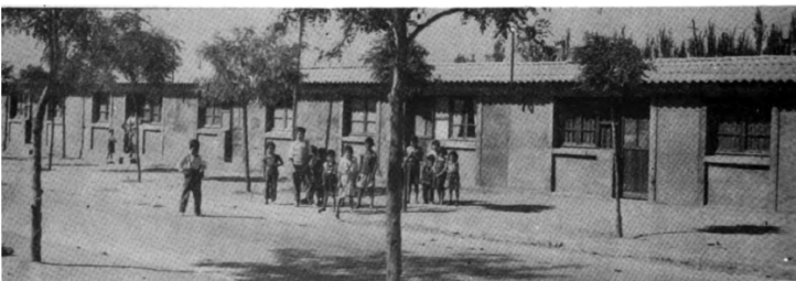
Figs.48-50 The Germán Riesco Aided Self-Help Housing Project, Santiago, Chile. Urban plan available at Lo Contador Library, Pontificia Universidad Católica de Chile. Photographs from Robinson, 'Chile's Solution', 36.
