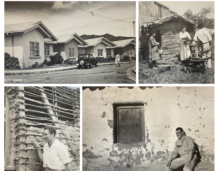
Figs.81-4 Costa Rica. (top) Government single-family housing project on the left, and Rafaela Espino conversing with occupants of an informal settlement on the right. (bottom) Bahareque constructions. The reverse of the photo on the right states: 'Len Currie in front of a bahareque house, approximately 125 years old.' Source: (top left and right) Box 1 Folder 11, (bottom left) Box 1 Folder 14, (bottom right) Box 1 Folder 15, VTECH
