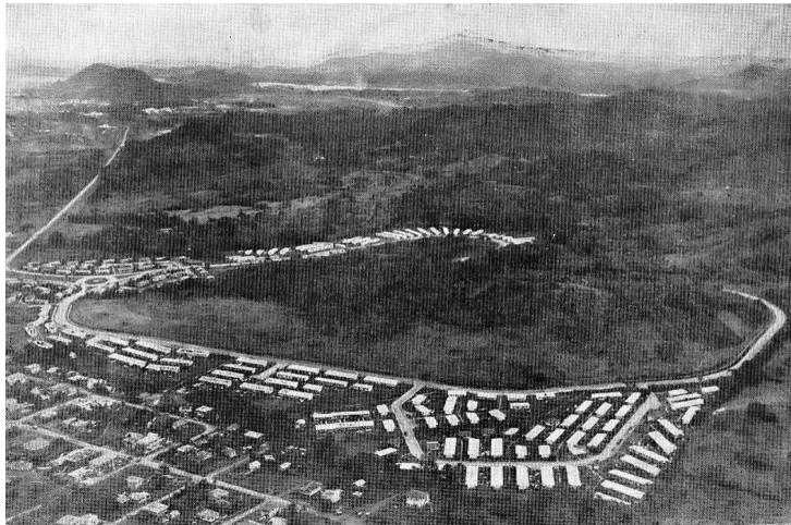
Fig.36 Vista Hermosa in construction, 1949 in Rubio, La Ciudad de Panamá , 101 reproduced in www.panurbis.wordpress.com/2021/09/08/betania/ Accessed May 13, 2023.
