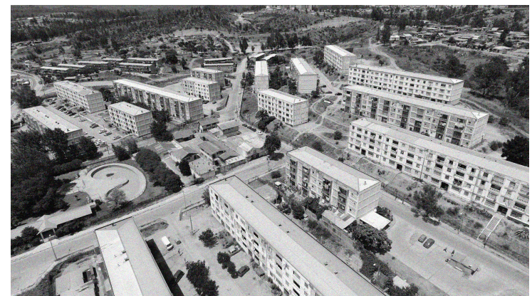
Figs.70-4 (top and middle) (top and middle) KPD Factory for prefabricated panel housing in Chile. Construction of the El Belloto neighbourhood in the Valparaíso region. Source: Corporación de la Vivienda, Planta KPD . (bottom) (bottom) El Belloto neighbourhood with the constructed multifamily housing buildings. Source: 'Reportaje del programa Frutos del País sobre El Belloto', El Belloto Comuna, 6 October 2016, http://www.elbellotocomuna.cl/2016/10/reportaje-del-programa-frutos-del-pais.html .
