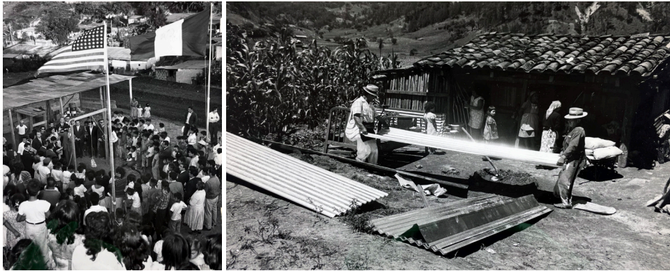
Figs.15-6 Alliance for Progress school and housing project in Guatemala. Source: Box 5, RG286-CF, Photographs from the Country Files ca. 1961 – ca. 2002, NARA.
