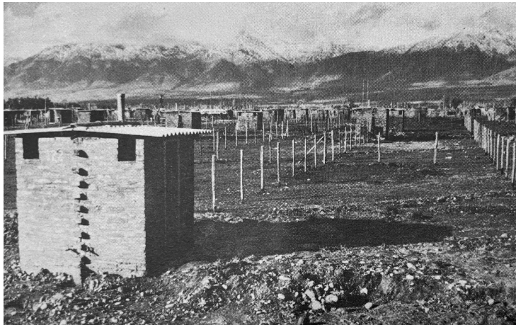
Fig.1: Initial stages of the San Gregorio housing project in Santiago de Chile, showing the plot demarcated with stakes and a sanitary core built at the rear of the site, with the Andes mountain range visible in the background. Source: Corporación de la Vivienda, Chile 1960 , 14.
