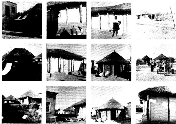
FRANCISTOWN: TATITOWN TRADITIONAL HOUSING – A PART OF THE FRANCISTOWN URBAN DEVELOPMENT PROJECT
