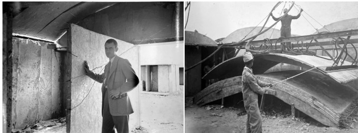
Figs.68-72 Leonard Curry in a house in Quiroga. Construction of Quiroga, Quiroga neighbourhood. Sources: (this page) Box 1 Folder 16, VTECH. (opposite page) Currie, Leonard J. (Leonard James), 1913-1996 (Photographer), "Unidad Vecinal (Community Housing Project) Quiroga, Bogotá," Southwest Virginia Digital Archive, accessed November 17, 2023, https://di.lib.vt.edu/items/show/484 .
