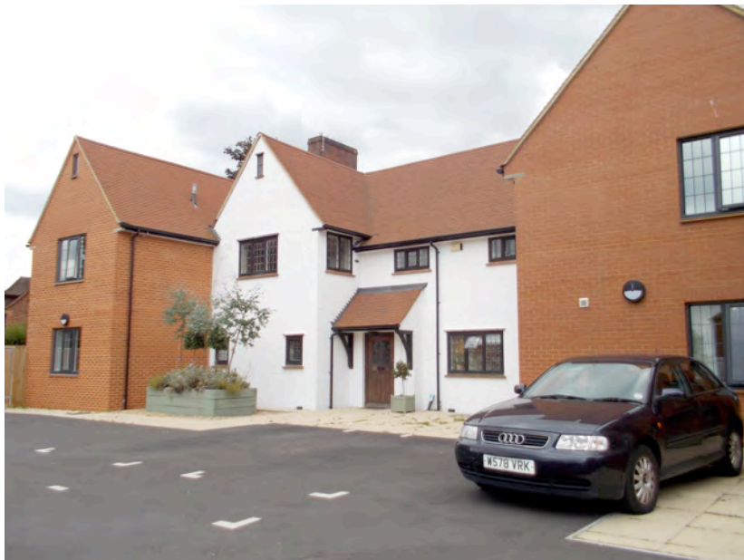
Figure 73. Kingwood College with White Barn next door (left)
