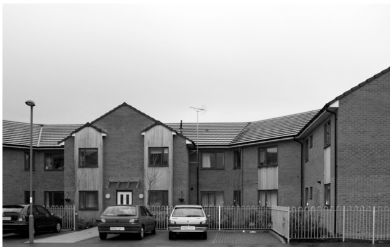
Figure 52. Exterior of Beeching Way
