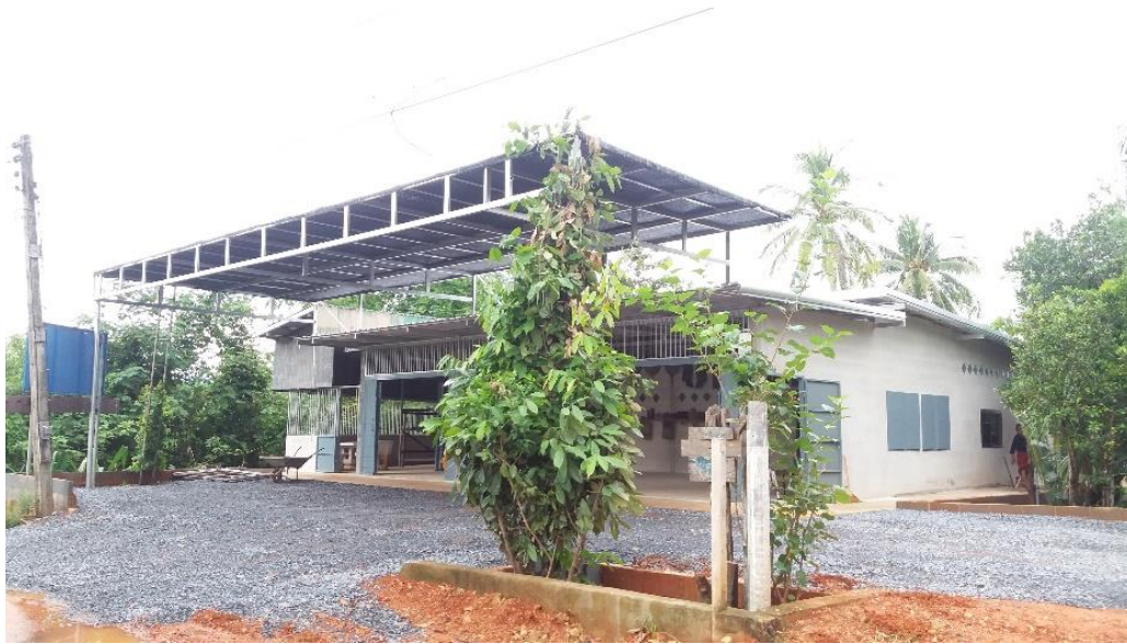
Picture 62. The front view of the house and weaving space after its renovation. Wuthigrai Siriphon, 2017.
